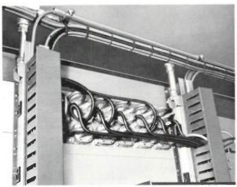
Figure 6: Directional Couplers Rack-Mounted for 12-Channel Head-End.
