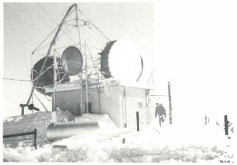
Five feet of snow blocked the entrance to the head-end building. Also note the bent mast of the 465 MHz microwave antenna which almost touches the ground.
