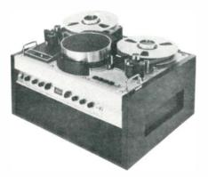
separately. The units accept any EIA signal, are compatible with all cameras and existing TV equipment, according to the manufacturer, and all feature stop-action. The DP-2 and DP-3 both offer 350-line resolution and are designed with removeable circuit modules and dual capstan drive. Both units utilize a rotary two-head system and 1-inch tape.
