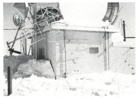
The storm on Pinal Peak near Globe, Arizona left the cable system's antennas strewn around the head-end site. The channel 12 antenna appears to be vertically polarized!
