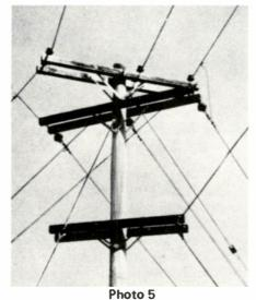
brace, radiates a very strong signal in the VHF band due to the length of the brace. By replacing the lag in the pole with a bolt and a nut on both sides, the brace is made solid. This same thing can be done with the bolts on the arm.
