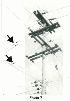
guys coming in contact with the cable system by touching the bare shield of the cable will also cause induced interference in the system. This contact, when ahead of the amplifier, can be a source of trouble, especially near the head-end.
