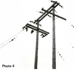
caused by dead ends on the 13kV insulators and slack guy cables. These are in an area of high corrosion near a smelter which also causes harmonics from the rectified arcing.
