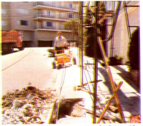
The boring head has been started in the soil. The guide tool, has been removed to show detail.
