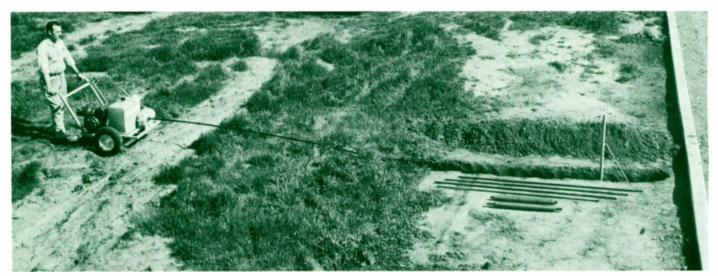
The compacting auger operation is shown in progress here. After the bore is completed, coaxial cable or conduit can be installed by swivel attached to reamer on return pass, or cable can be hand fed through the bore.
