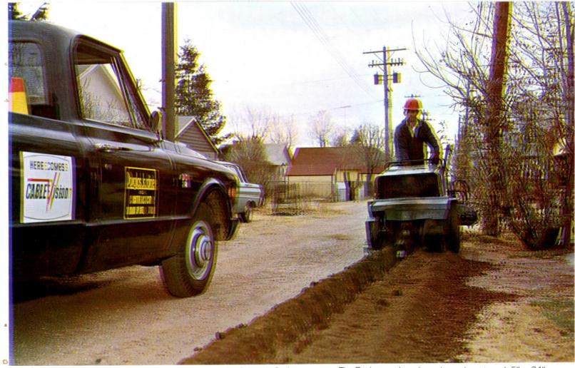
Dver 400 miles on underground plant make up the Colorado Springs system. The Davis trencher shown is cutting a trench 5" x 24".
