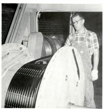
Charles Bolick guides first traverse of 3/4" Alumagard onto 2000 ft. reel. Cable on reels in background will receive the same jacketing. Flame treating sets sequential footage and identification markings.
