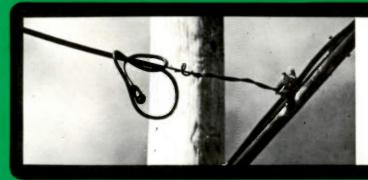
Disconnected drops like this invite cheaters to hook up the connections for free service. The openings to the main cable and the house line let water seep in thus causing damage.
