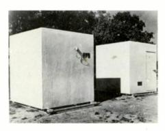
are available for each custom-assembled building. They include air conditioning, exterior lighting, electrical outlets and lighting units, partitions, toilet and plumbing facilities, battery cabinets, louvers and exhaust fans. Company colors may be applied to the building during its fiberglassing and company emblems and numbers can be built into the exterior walls.
