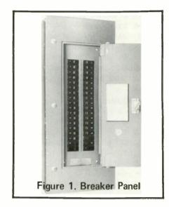
because most panels are usually located away from the production area. The breaker panel has the advantage of low initial cost.
