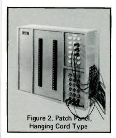
must be done when installing the dimming system is the re-routing of prime power to the dimmer bank, connection of dimmer bank to patch panel and connection to control console. Financially, this represents a greater initial investment than the breaker panel, but
