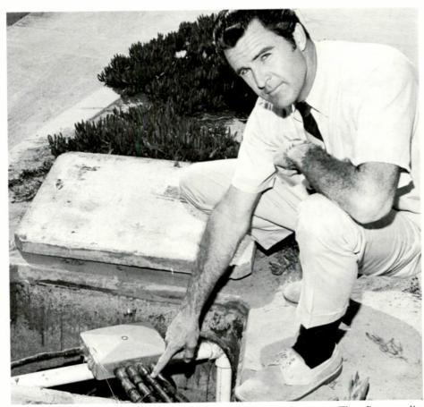
Underground construction is becoming increasingly popular. The Community Cablevision system at Irvine, California is totally underground. System manager Gene Moon is shown here checking moisture-proofing of an amplifier in a vault. Approximately 50% of all California immigrants move into Orange County... and a high percentage of these people will eventually settle in the 83,000-acre "master-planned" City of Irvine. See a special report on this system in May TVC.
