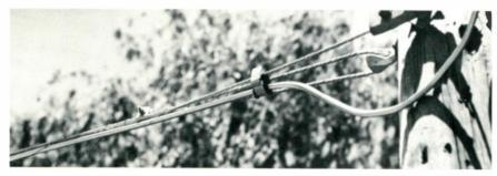
Preformed False Dead-End is used at guyed pole. Permits straight-through continuation of cable and messenger. Often used when a slack span is needed.
