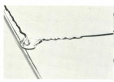
In some cases it is preferable to bring the service wire off the tap to a point somewhere in midspan where a neat connection is made with two Telegrips.
