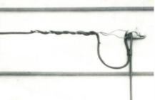
Telegrip is neatest way to bring service wire to the house entrance. It prevents kinks in the wire and helps give distortion-free picture.
