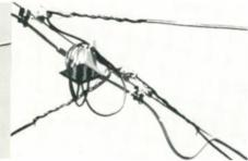
Three-way tap-off is made with Telegrips, which are connected to span clamps and carry the wire to the house.
