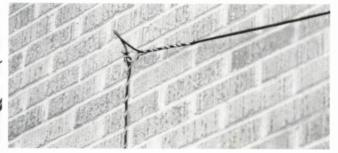
Two PREFORMED connectors are used to secure house drop cable. A firm but gentle grip prevents crushing or abraiding of cable.
