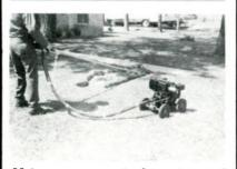
Using our swivel unit and special water bit will enable you to drill under driveways. The drill stem is standard 3/4" water pipe.
