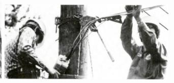
Messenger which supports feeder cable is tensioned with come-along prior to permanent attachment to pole fitting with PREFORMED GUY-GRIP® Dead-end.
