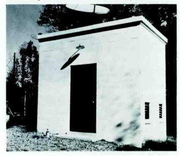
This is a good example of a well-built equipment building. Construction is of concrete block with reinforced louvers on the side. Also notice the heavy steel door.
