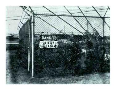
Fences like these around guy anchors will aid in preventing damage. Note the use of the "Danger-High Voltage" sign.
