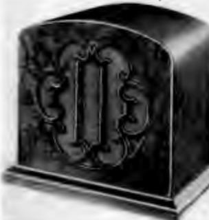
following models: Models 7-A, magnetic type speaker cabinet of Gothic design; 12 1/2" high at center; 11 1/2" at base, and 7" deep. Model 17-A, dynamic type speaker, mahogany cabinet; 14 1/2" high at center; 12 1/2" wide at base, and 9 1/4" deep at base. Model 19-A, dynamic type speaker, made of
