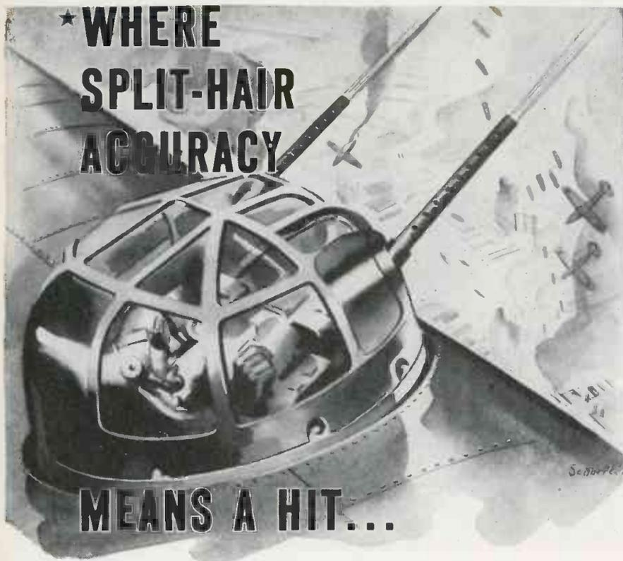
*Shown below is a Utah Potentiometer for power-driven machine gun or cannon aircraft turrets. This gunner has feather-touch control of his guns' position—no matter from which direction the enemy may attack. In this precision operation, the Utah part plays a vital role. It has been fitted for that role by split-hair accuracy in manufacture. This is only one of many Utah products now in service with the armed forces.*
