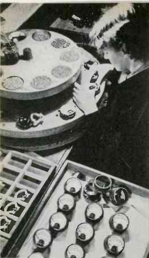
▲ "LAZY SUE" table at Newark, N. J. Weston plant speeds production instead of passing salt and pepper. Light touch on edge of top rotating table positions parts-cups in final assembly of instruments while lower table delivers sub-assemblies. Another turntable idea, top right, ups assembly of Westinghouse motors by 25%. Motor is placed on dolly over conveyor, worker rotates it to tighten all four feet before returning motor to conveyor belt
