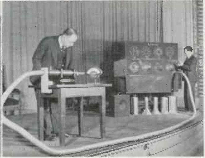
Above, Dr. Southworth is shown holding one of his resonant chambers used for wave-guide tests, while he stands in front of the two experimental wave-guide transmission lines at Holmdel, N. J. At the right Dr. Southworth is seen making a platform demonstration of uhf guided by tubing
