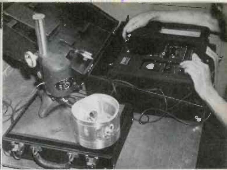
**SURFACE FINISH** check on piston pin hole for Wright Cyclone engine using Brush surface analyzer, at Paterson, N. J.
