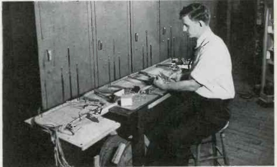
▲ **BLIND WORKER** at Link Radio Corp., N. Y., puts his delicate sense of touch to work fastening solderless connectors to intricate cable assemblies. Link has many blind workers who excel all others
