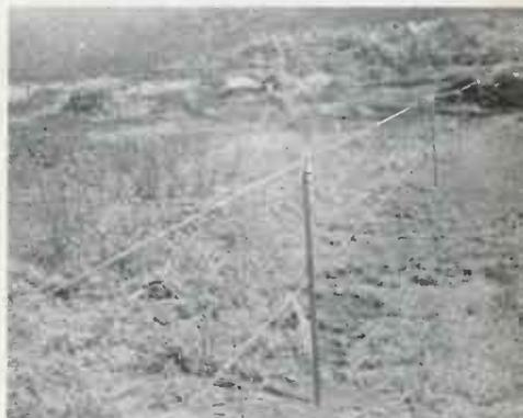
"Telapproach" wires of capacitance system
