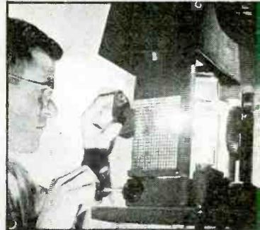
**METALLURGY**—*Spectrographic Analysis of the Rare Metals Used in Vacuum Tube*
