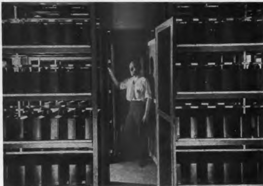
Bank of capacitors used to bring the power factor of the magnet energizing circuit up to unity. About 1,000 amperes are supplied and the resonant voltage is 4,000. Coils dissipate 120 kw
