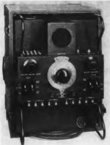
Fig. 1—Front view of Lookator unit with cover removed. Viewing tube is mounted over dial
