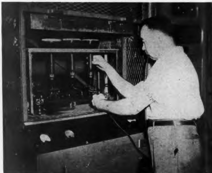
Fig. 14. "Sealing in", or connecting the glass of the stem to the bulb
