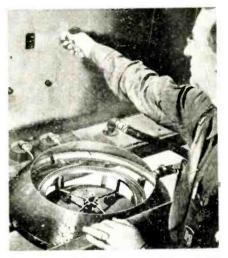
Ring gear ready for 20 sec. hardening operation
