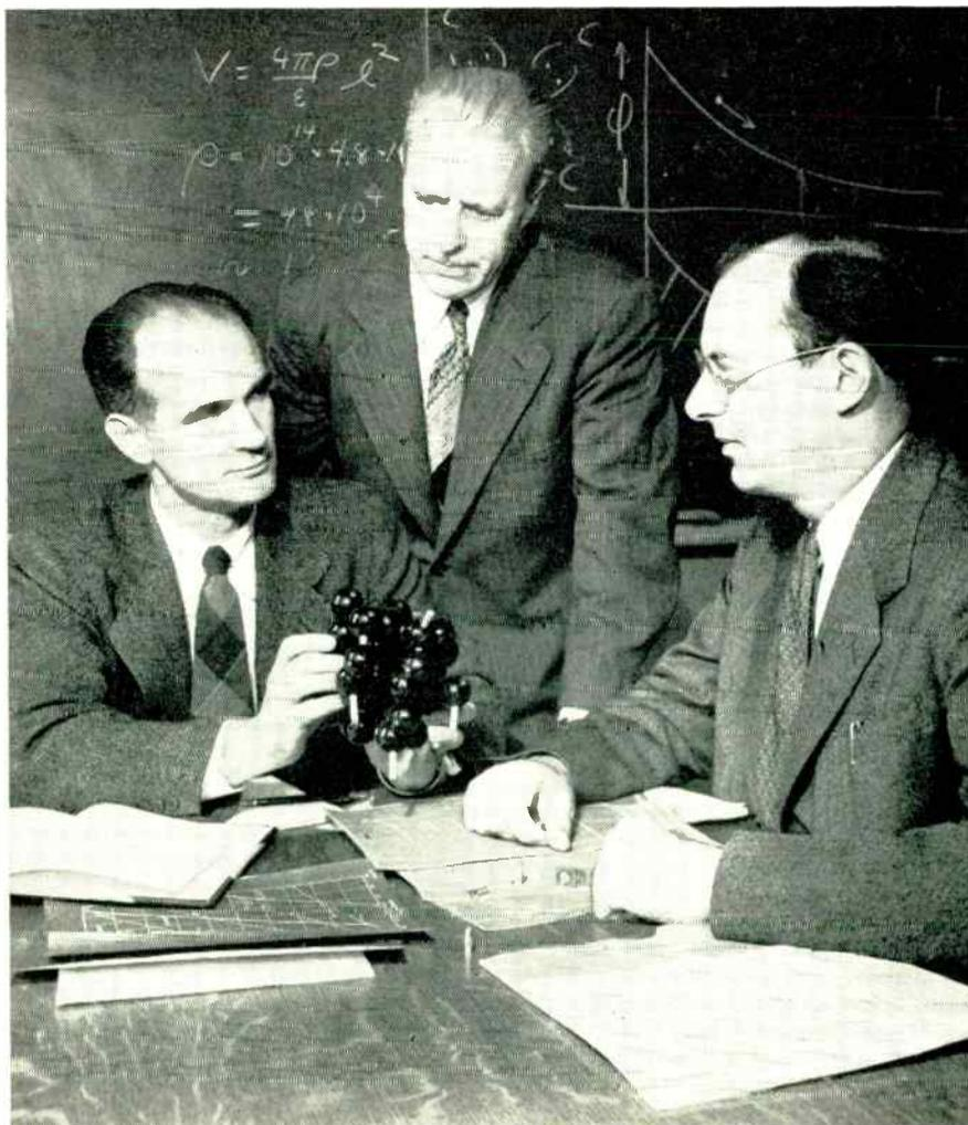
**Bell Lab demonstrates germanium crystal device which amplifies and oscillates. Inventors display tubeless radio receiver. Observers suggest transistor might replace some tubes in TV sets; industry comments pro and con**
