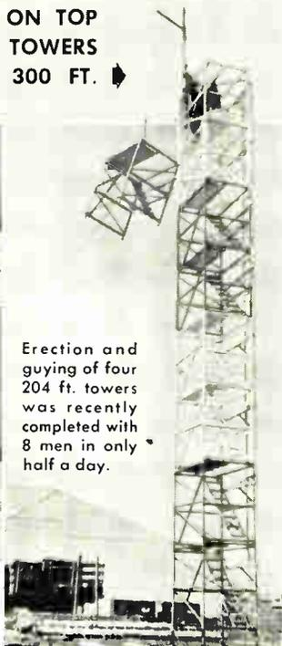
Erection and guying of four 204 ft. towers was recently completed with 8 men in only half a day.
