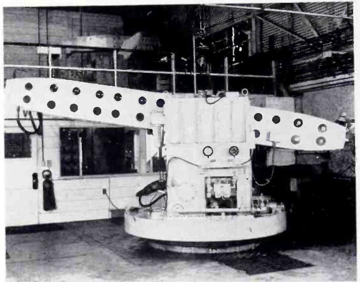
(Above) Hydrodynamic Simulator at Naval Ordnance Test Station, Pasadena, Calif., tests torpedoes under simulated sea environment.
