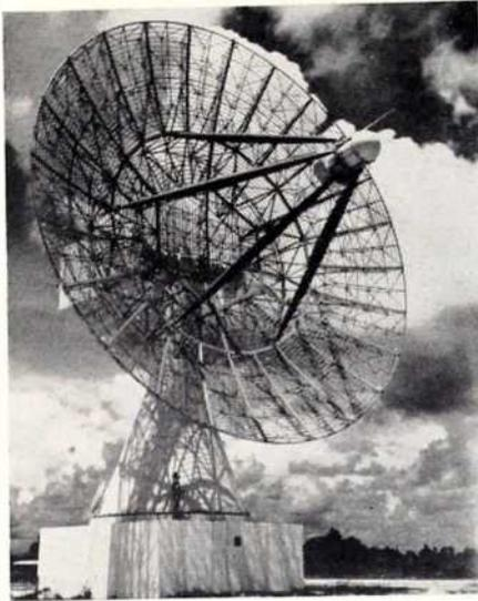
Higher than a 7-story building this giant 60-ft wide antenna built for ARDC by Radiation Inc. at Melbourne, Fla., is one of five that will pick up telemetering information from highflying-ballistic missiles.
