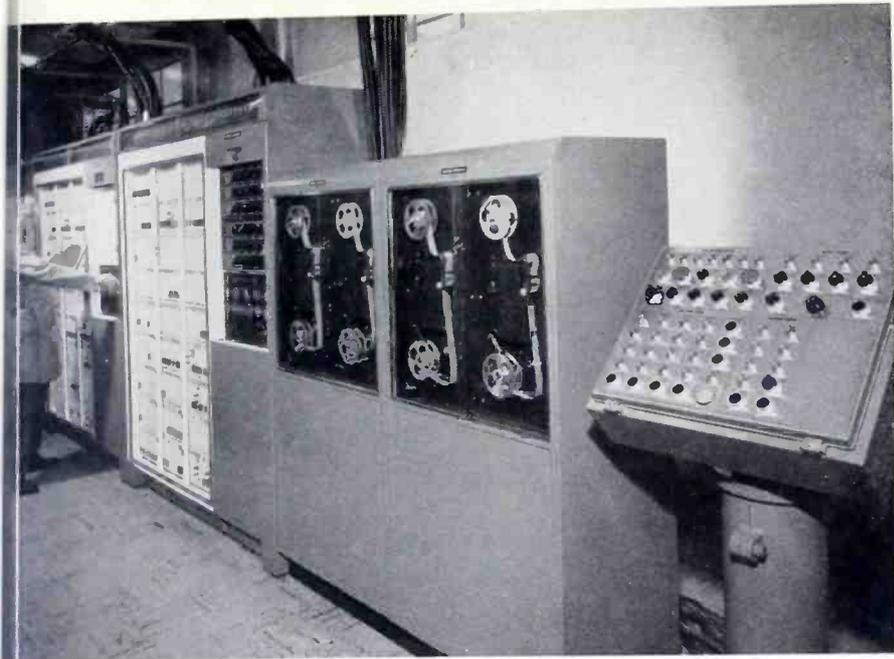
Fig 4: This is the electronic "Digitape" nerve center of the electronically controlled machine. Norman Wells, Hughes research assistant, checks drilling control cabinet.
