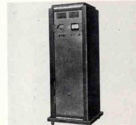
CPS, output voltage 0-130 volts, single phase, 2KVA. Input is 230 volts 60 CPS, single phase. Behlman Engineering Co., 2911 Winona Ave., Burbank, Calif.
