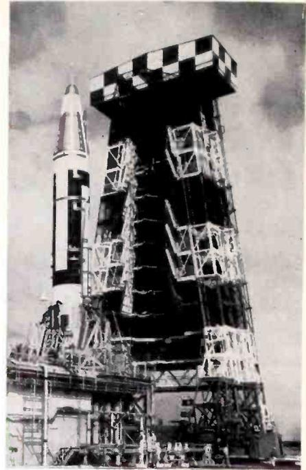
Gantry tower used in readying the Atlas ICBM is rolled away from launch stand, leaving missile poised for flight, at the AFMTC, Cape Canaveral, Fla. Convair-Astronautics designed and built the Atlas.
