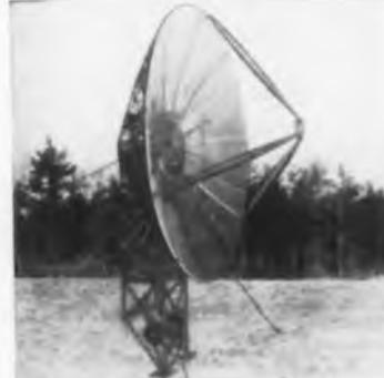
tower are used to convert the structure into a trailer which can be towed over public highways or difficult terrain. Adapts particularly to scatter propagation site surveys. It may be rolled aboard a military transport plane and secured without additional crating. Known as Model 749, it is adaptable for use between 200 and 4000 MC. D. S. Kennedy & Co., Cohasset, Mass.
