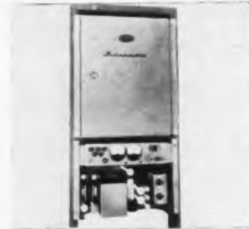
izer. Portable version is housed in 4 rugged, lightweight cases. Broadband waveguide plumbing allows operation from 5925 to 7425 MC. Raytheon Mfg. Co., Waltham, Mass.
