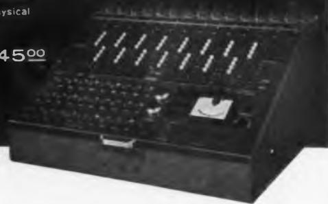
This advanced "slide-rule" is a highly accurate device that permits engineering or research personnel to simulate equations or physical problems electronically, and save many hours of involved calculation.
