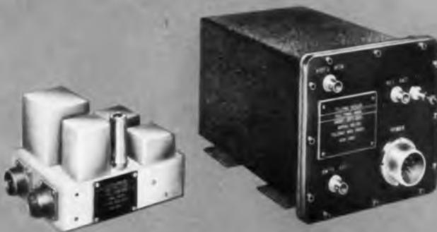
New superheterodyne S-Band Beacons for guided missile and drone-control applications. These receivers feature light weight, small size, excellent reliability, ruggedized construction.
