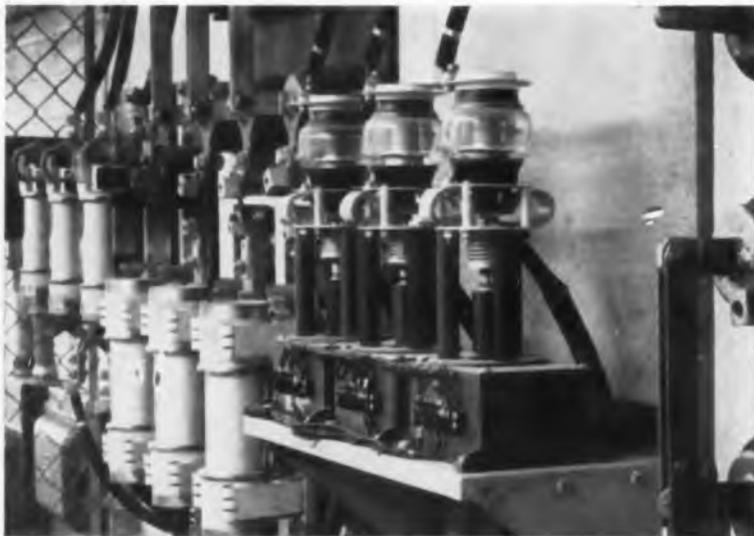
2400 volt overload protection for General Electric's new 50kw broadcast transmitter in service at station XEAK Tijuana, Mexico.
