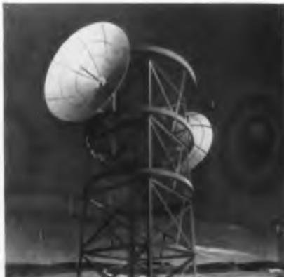
Ring mounts simplify orientation, make future antenna installation easier and less costly.
