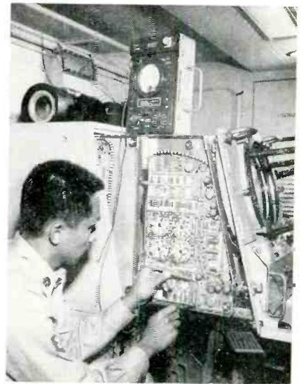
Entire console section (above) of 3-dimensional radar slides out on rollers for easy testing and quick replacement of parts.
