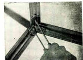
Locking connector and extrusions
