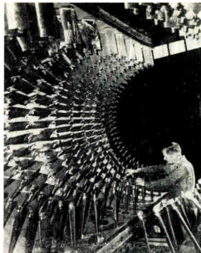
Auxiliary compressor designed by Westinghouse for the 16 ft. transonic wind tunnel at NASA, Langley Field, Va. will remove dead air around tunnel at 1,000,000 ft 3 min.
