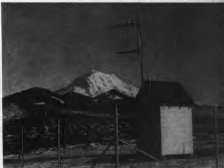
Depth of snow on remote mountainsides is being continuously reported by FM radio through this Motorola transmitting station. Radio-active metals at ground level activate Geiger counters suspended above maximum snow height. Presence of the snow cuts off radiation reaching counter proportionally to depth and water content of snow pack. In this way an accurate measurement of future melt can be reported to water users in valleys below.
