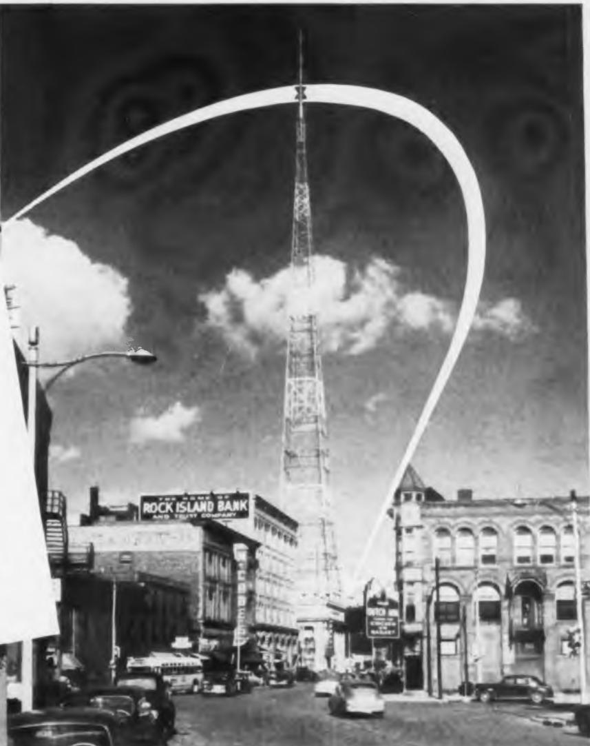
*WHBF's TV tower, with an overall height of 182 ft., was mounted on a specially constructed substructure 61 ft. high. Tower is designed to mount station call letters on all 4 sides, and carries an RCA custom-built, 5-section, Super Turnstile antenna.*
