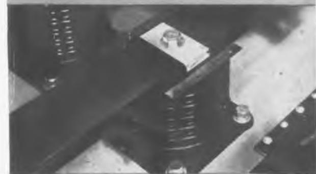
Bus support with and without Phenolite insulating covers.
