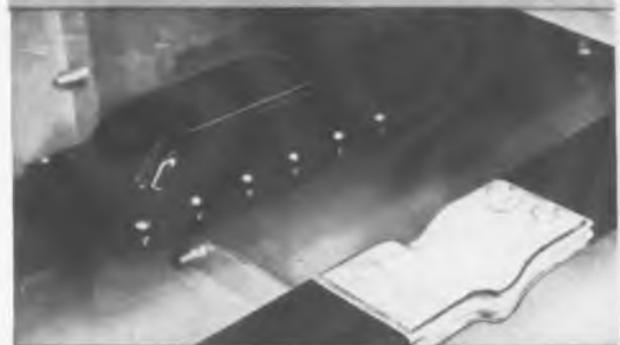
Expansion joint with and without Phenolite insulating covers
