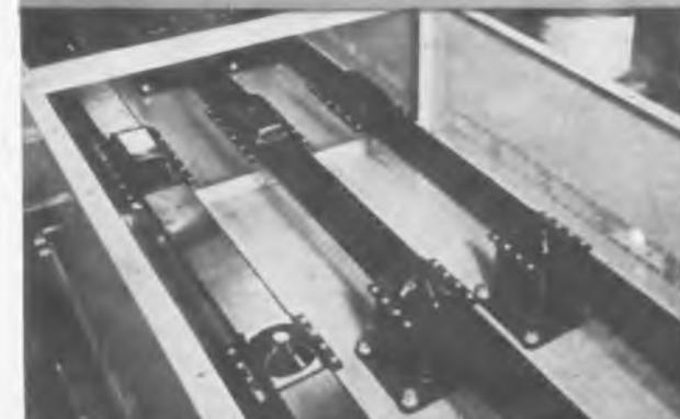
Completed installation, showing Phenolite insulation for bus bars, supports and expansion joints.
