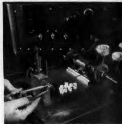
Fig. 8: Cores of Hiperthin  $\frac{1}{2}$ -mil steel are wound on ceramic spools and then spot-welded
