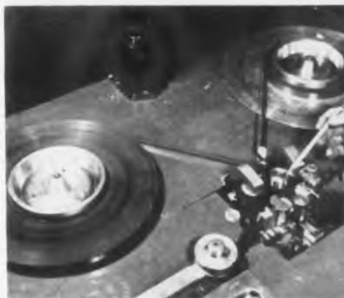
Fig. 3: Tape drive mechanism
