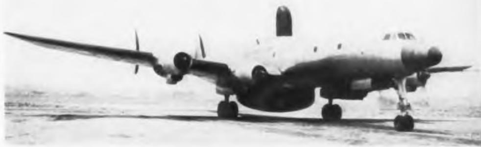
Fig. 4: Flying radar station with bulging radomes is part of extra-early warning system
