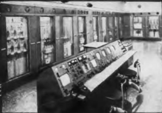
Transmitter room at WOR-TV's new Empire State 50 KW transmitter, 130 KW ERP, 100% air cooled. Completely self-contained. Equipment throughout by Standard Electronics.
