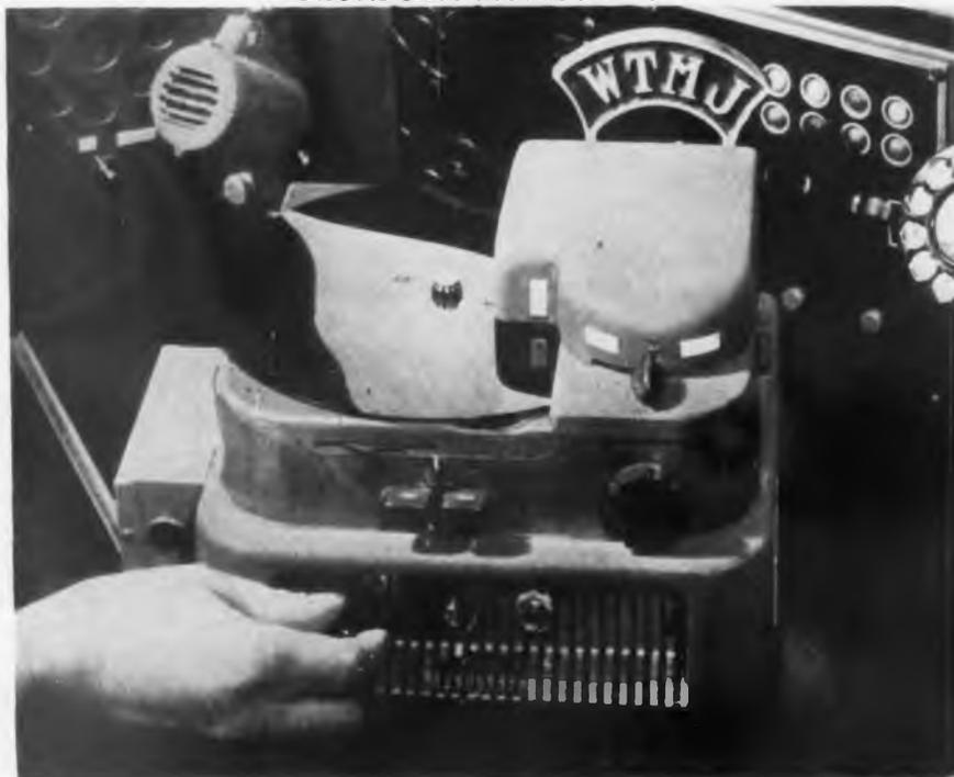
Here is how Station WTMJ, Milwaukee, Wis., keeps an air check of all shows going out over the airwaves from its broadcasting station. Broadcasts are monitored on an Audograph. Paper-thin plastic disc records clearly and economically a full half-hour show on each side. A hundred hours of broadcasting can be permanently recorded and filed in a box only an inch and a half deep and nine in. sq.
