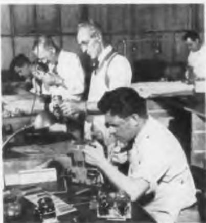
**3** The assembly of precision units machined to within 0.0005 in. requires skilled workmanship. Here, jeweler's glass aids delicate adjustment of Computer section
