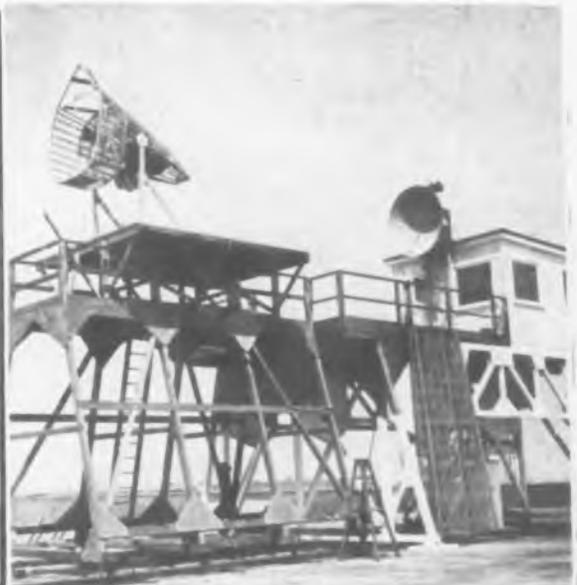
Fig. 9: (l) Method of providing access to hollow interior. Silver plated beryllium copper strip provides leak-free contact between shell sections. Fig. 10: (r) Douglas Aircraft's antenna range has elevated structure to minimize ground reflections. Nose section shown is movable along track
