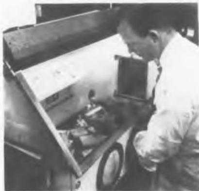
Bell Labs engineer uses "dry box" to assemble new UHF transistor. He is shown placing casing over transistor. Units operate at 440 mc
