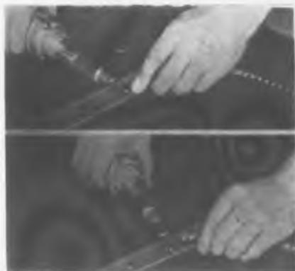
terchangeable for number 6-8-10 and 14Z screws. The fasteners are in coils or strips of any desired length and designed for making power-driven attachments with type A or B (Z) sheet metal screws. Provide double-locking, vibration-free attachments. The operator merely positions the nut end and power-drives a screw. A slight hand pressure snaps the nut from the strip. **Tinnerman Products, Inc., P. O. Box 6688, Cleveland, O.—TELE-TECH & ELECTRONIC INDUSTRIES.**
