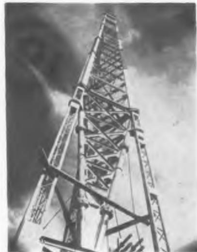
The 1572 foot tower, a triangular guyed structure, measures 12 feet in width across each of its three faces. It is supported by a total of 24 guy cables spanning out to anchors almost a fifth of a mile from the base. Total weight of the massive structure will be over 1,300,000 pounds.
