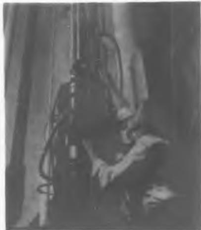
First photo of 4-megawatt klystron designed for high power Air Force radar. The 8-ft. tall tube is shown being installed at Rome ADC, N. Y.
