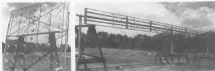
Extension of UHF-TV service into areas blacked out because of geographic conditions has been proved feasible, according to field tests conducted by RCA in conjunction with WJTV, Jackson, Miss. Booster equipment installed 37 miles from the transmitter stepped up field intensities 23 db to Grade A service. At left is 8-ft. sq. receiving antenna with power gain of 100. At right is 38-ft. transmitting antenna with power gain of 100 which transmitted 10 watts from booster amplifier
