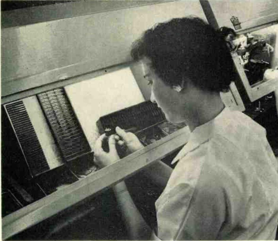
Cage Assembly, the first step in mounting tubes is performed under hoods. The operator, dressed in the required white lintless uniform, is wearing rubber cots on each finger to protect the mount from moisture.
