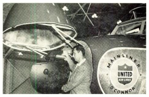
United Air Lines exec. demonstrates operation of C-Band radar
