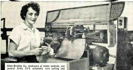
Allen-Bradley Co., producers of motor controls, use several Artos CS-6 automatic wire cutting and stripping machines in their Milwaukee plant.
