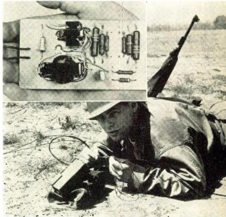
Signal Corps technician splices the new transistorized repeater into field telephone line. New unit, thanks to transistor, and use of printed circuit construction, is only 1/5th the size and weight of the wartime version. Batteries last 90 days, and cost \$6.00 yearly. Batteries for similar WW II model cost \$105 yearly. Predicted field life of the new repeater is 10 to 15 yrs.—without adjustment.
