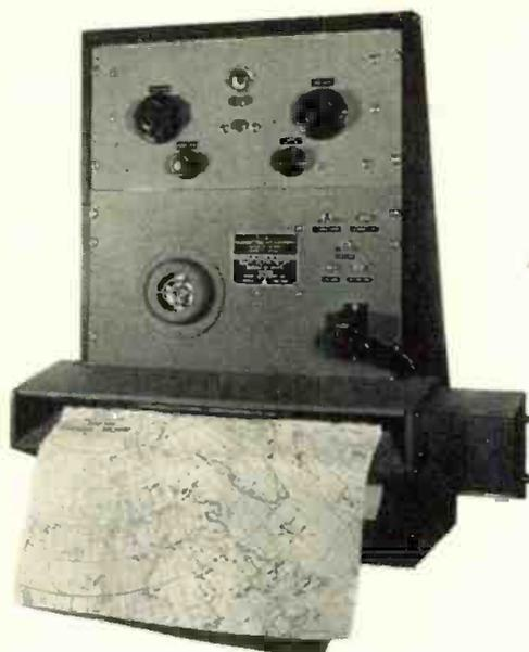
Fig. 1: The X-1x Facsimile Transmitter with weather map feeding past scan line
