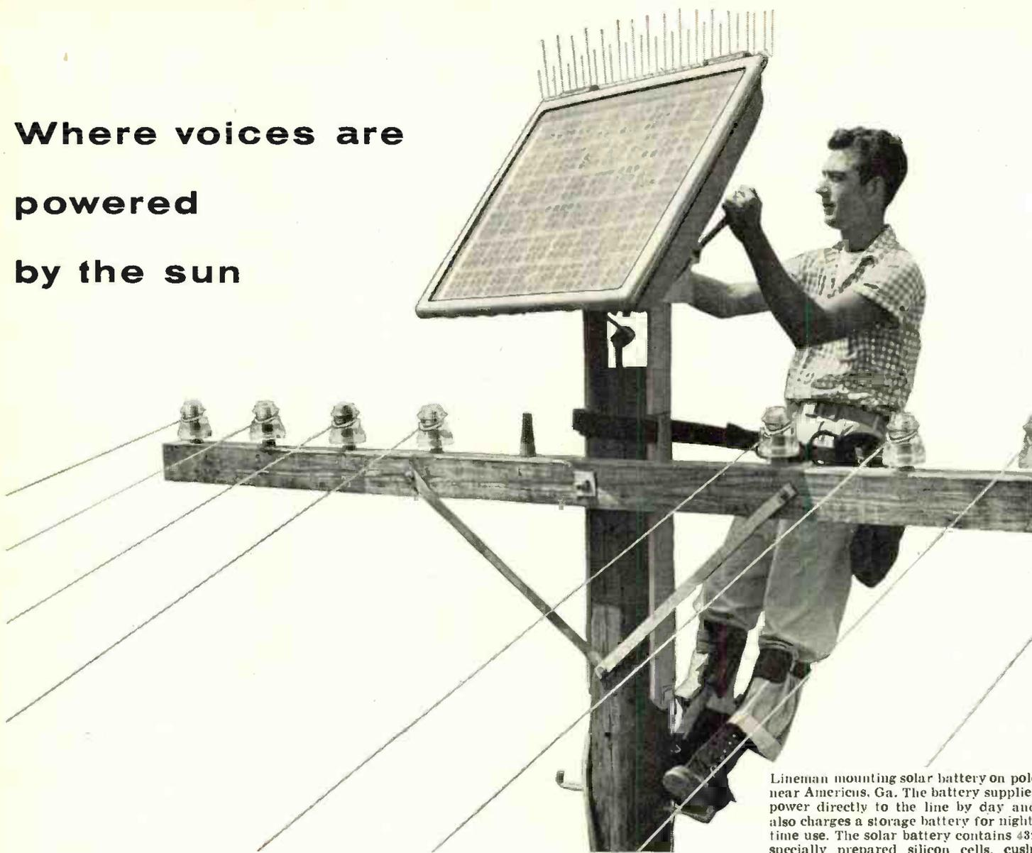
Lineman mounting solar battery on pole near Americus, Ga. The battery supplies power directly to the line by day and also charges a storage battery for nighttime use. The solar battery contains 432 specially prepared silicon cells, cushioned in oil and covered by glass.
