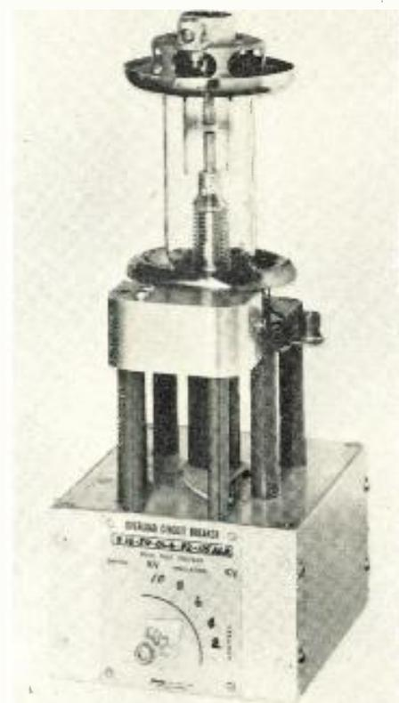
Fig. 9: 5 millisecc overload circuit breaker using  $\frac{1}{4}$  in. diameter contacts of 50 kv test
