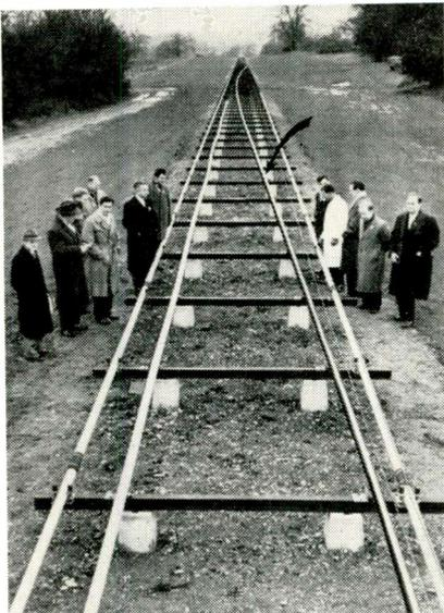
IT&T Corp. is sending live TV over half a mile through this 3 in. pipe at Hertfordshire County, England. They are believed to be the first transmitted by circular waveguide or by pulse code modulation for such a distance. Even greater distances are possible with repeaters. In commercial use, the pipe would be buried.
