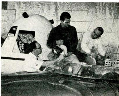
A biomedical instrumentation system designed to flash the physical and emotional reactions of spacemen back to earth is tested in this racing car at Riverside, Calif. System was developed by Norair Div., Northrop Corp. Hawthorne, California. Northrop Corp's space capsule mock-up is in the background.
