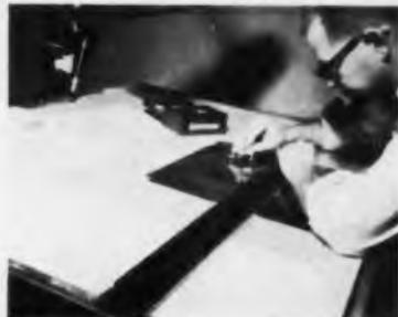
Fig. 2. Mr. Saude peels out circuit path by lifting one edge of film in the outlined area and pulling it from sheet.
