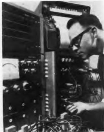
Minutes equal months on this analog computer used by Minneapolis-Honeywell temperature engineers to duplicate climate and building conditions anywhere in the world. Research engineer Donald Nelson can obtain in 15 minutes technical data that would normally take years to assemble. It is used to evaluate performance capabilities of new temperature controls.
