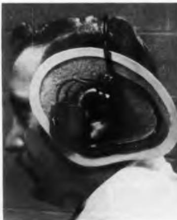
Fig. 3: An "earful" of essential medical information is provided by the "clothespin" type transducer clipped to the ear of this hospital patient. It measures diastolic and systolic blood pressure and pulse rate by shining a light through the patient's ear onto a photocell.
