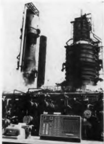
American Oil Co. has installed a fully automatic, closed-loop, process control system developed by IBM at its 140,000-barrel-a-day crude oil distillation unit, at Whiting, Ind. The control system which will continuously monitor and control the crude unit is built around an IBM 1720 Solid-State Digital computer.
