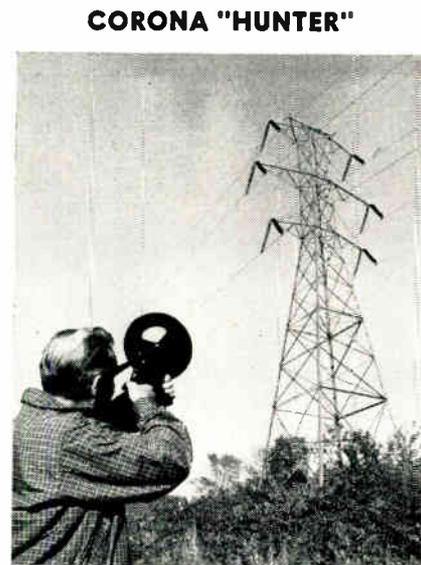
Aiming an ultrasonic "gun" at a high-voltage transmission line, W. E. Pakala of the Westinghouse research labs tests the line for electrical leakage, or corona. If present, corona produces high-frequency sound waves which are received by the "gun" and made audible through electronic circuitry. A telescopic rifle sight built into the instrument pinpoints the corona sources.
