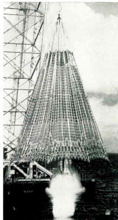
Set up off the coast of California, huge "grab-bag" catches a 15-ton test vehicle as it breaks the surface after being launched from a tube on the ocean's floor. Special draw strings snap the bag shut as the *Polaris* enters. This enables Lockheed Missiles & Space Co. engineers to study missile's underwater performance, and prevents damage to the "sea-bird," permitting repeated use of the test vehicle.
