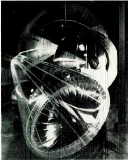
Inflatable space structure is the prototype of a new rigidized solar collector able to serve as a satellite or space vehicle piggy-back power generating device. Developed by Viron, a division of Geophysics Corp. of America, Bedford, Mass., is designed to be inflated outside of a satellite or space vehicle. Other inflatable structures in the background are plastic balloons built for use as ground, air, and rocket-launched target spheres.
