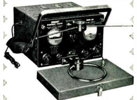
This versatile instrument is a highly sensitive interference locator—with the widest frequency range of any standard available unit! Model 500 tunes across the entire standard and FM broadcast, shortwave, and VHF-TV spectrums from 550 kc. to 220 mc. in 6 bands.
