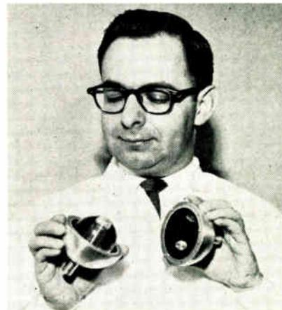
All-pneumatic gyroscope for space navigation is shown by G. S. Spleen, physicist of ITT Federal Laboratories, which developed it. Crystal ball supported by air cushion spins on fixed axis inside second sphere. Spheres turn at same speed, but independently. Drift is small since air cushion is nearly frictionless.
