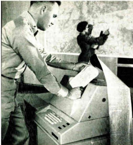
Fig. 4. Lt. A. Clum operates U.S. Army teleprinter. The general-purpose message printer can type at 3,000 words/min.
