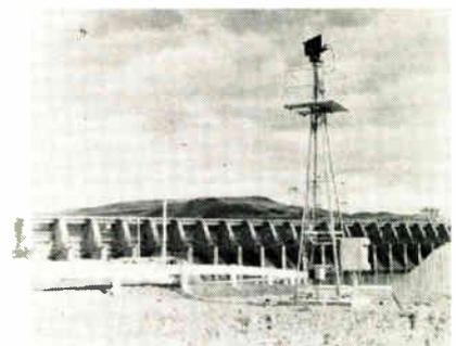
This camera is part of a 4-camera closed circuit TV system at Dalles Dam in Oregon. System "looks out" for log jams, ice floes, and other hazards in the reservoir. Manufactured by the Dage Div. of Thompson Ramo Wooldridge Inc., for the U. S. Army Corps of Engineers, the entire surveillance and security TV system operates round-the-clock in all weather conditions.
