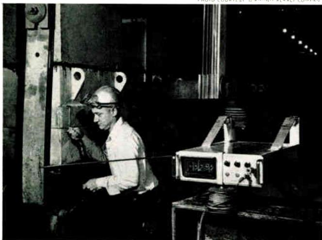
*Digital voltmeter is used to detect small voltage drops.*
