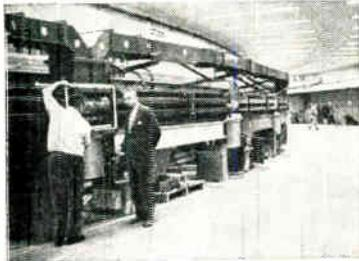
The Cambridge Electron Accelerator is an electron synchrotron of the alternating gradient type designed to deliver approximately  $6 \times 10^{12}$  electrons per second at 6 Bev. The electrons acquire this energy while executing 10,000 turns around the circular orbit. When directed into the 100' x 300' experimental hall, their mass is about 12,000 times the rest mass, and their speed is 0.999,999,99 times the speed of light in vacuum.
