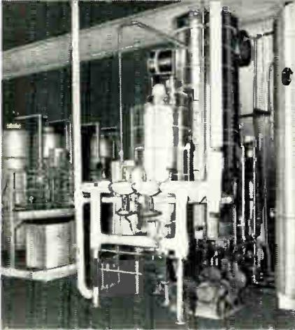
Above: Barnstead Double-Effect High Purity Still, Barnstead Four-Bed Demineralizer for pre-treatment of raw water installed at Sperry Rand Semi-Conductor Division, Norwalk, Conn.
