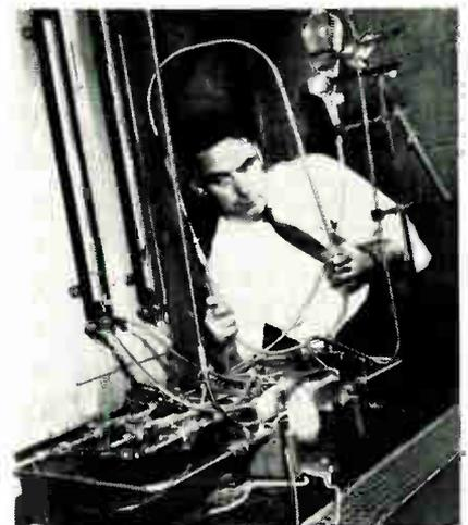
Mercury circulated through this tubing creates a force which G.E. says can be used to solve the problem of how to stabilize space vehicles on long flights away from earth. Normally, spacecraft are stabilized by jets expelling fuel in a direction opposite the erratic movement. Engineer R. E. Tompkins assembles a development model of the "fluid flywheel" at company's lab.
