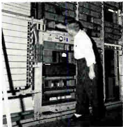
In Chardon, Ohio, near Cleveland, engineer inspects Stromberg-Carlson Register-Sender. It can be gradually integrated with existing electro-mechanical equipment to provide electronic switching advantages, including push-button dialing.
