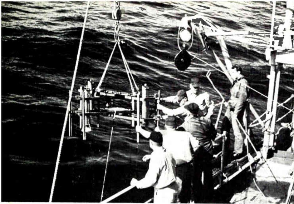
Underwater camera system with electronic controls, developed by Edgerton, Germeshausen & Grier, coming out of the water.
