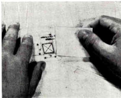
This backing sheet will be used on all Stanpat preprinted repetitive symbols and drawing details. The backing sheet lays flat regardless of atmospheric conditions. It is transparent, allowing draftsmen to position the Stanpat before application to drawing. Without any change to the adhesive, both sides of the sheet are now sealed to prevent any absorption of moisture. Stanpat Products Inc., Whitestone, N. Y.
