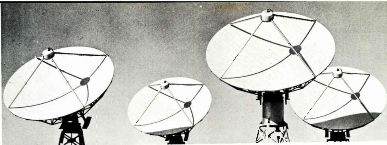
Fig. 2: Multi-reflector systems offer a method for antenna gains in excess of that possible from single apertures.
