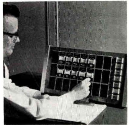
Standardized remote-control system called Conitel 10 for general industrial use can control and supervise up to 24 devices, which operate field equipment such as circuit breakers, valves and pumps. Designed by General Telephone & Electronics, the system can operate over any communications media.
