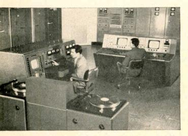
WOR TV engineers Frank Garufy and James Long (l. to r.) operate TV signal in the transmitter building. Foreground equipment is "sound desk" for playing records. Cabinets in background hold reserve transmitter equipment for replacements and emergencies
