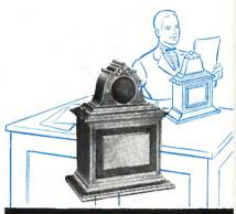
1921: The condensor microphone, designed by Bell Laboratories for sound measurement in 1916, entered the public address and broadcasting fields. It provided a wide frequency range and reduced distortion.
