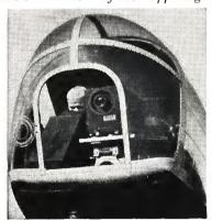
A television "eye" in the nose of a plane! Besides covering news events by plane, automobile or boat, such revolutionary equipment developed by RCA and NBC, can make accurate geographical surveys from planes flown by remote control. Moreover, similar television equipment can observe hazardous manufacturing processes from a safe distance.
