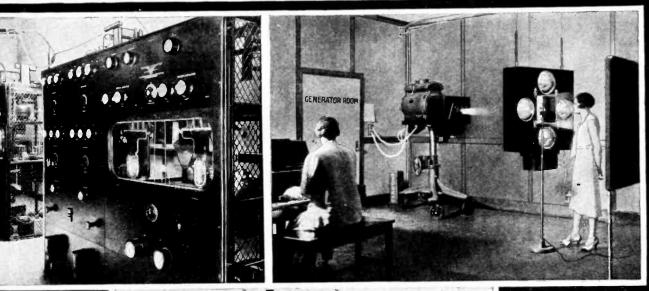
Above—The two transmit-ters at Roston; the further one, WIXAU, transmits rolee with 500 watts on 1.550 k.c. The one in the foreground, WIX.W. sated or 3.000 watts, on a frequency of 1.600-1.700 k.e. There is also an ultra-short wave transmitter,
