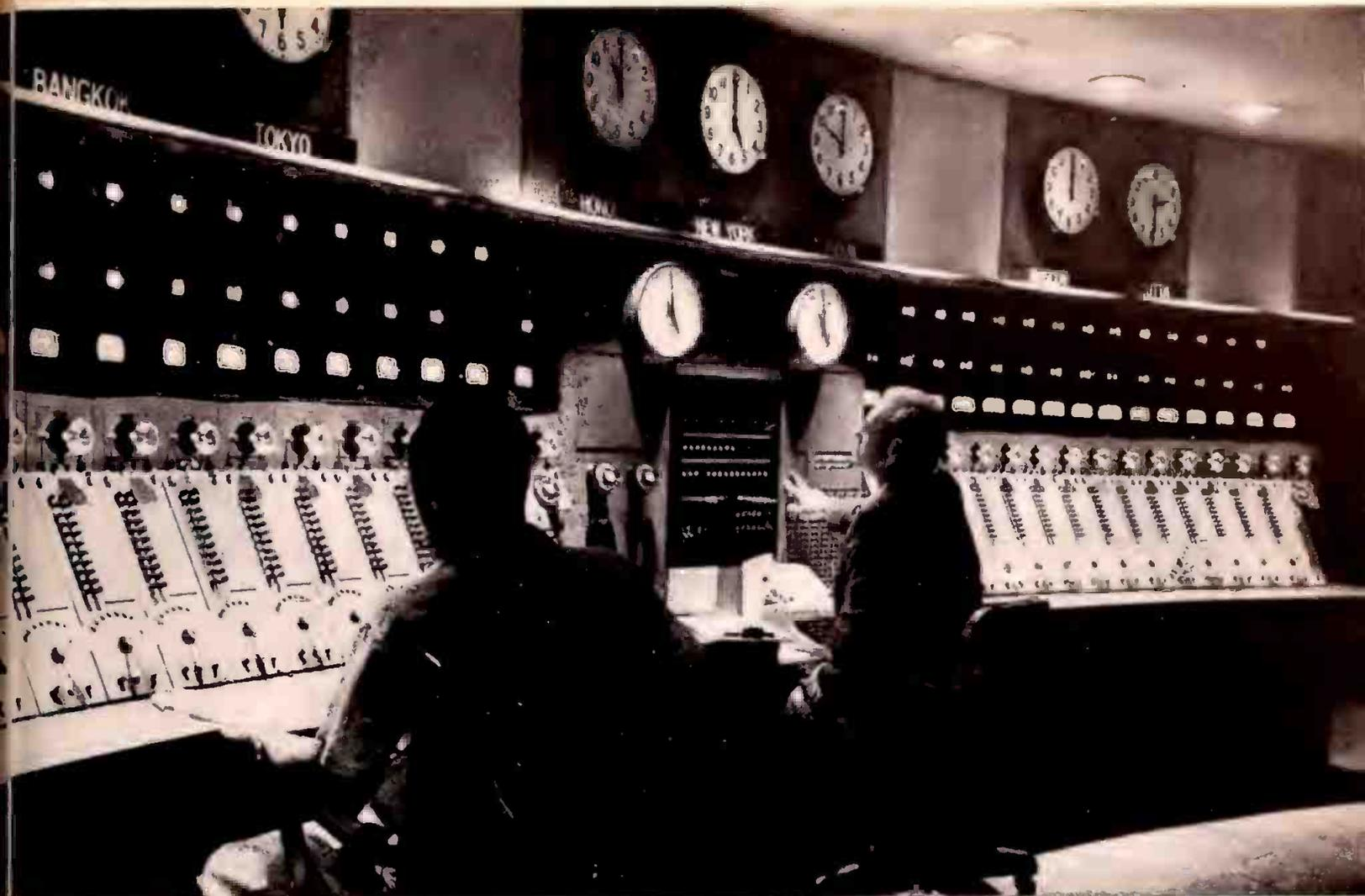
MASTER CONTROL console can select programs from 100 different sources and transmit 26 programs simultaneously. It is manned by two technicians at all times. Clocks tell international time.
