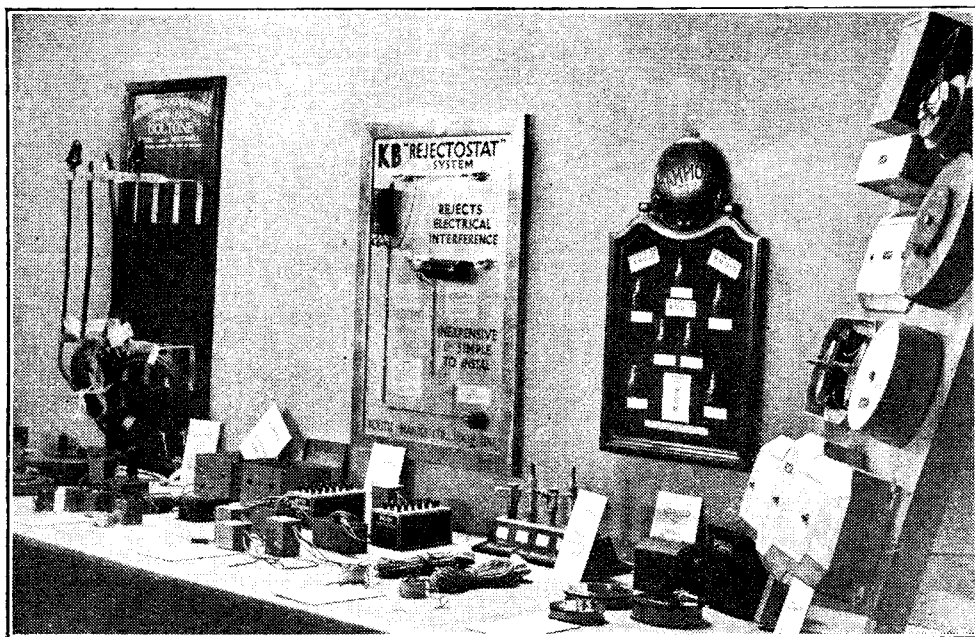
An interesting corner of the Post Office "village," showing various anti-interference devices lent by the leading firms.
