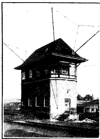
RAILWAY RADIO. A peculiar roof aerial on a German State Railways signal box at Herford. Train shunting instructions are transmitted on ultra-short waves.
