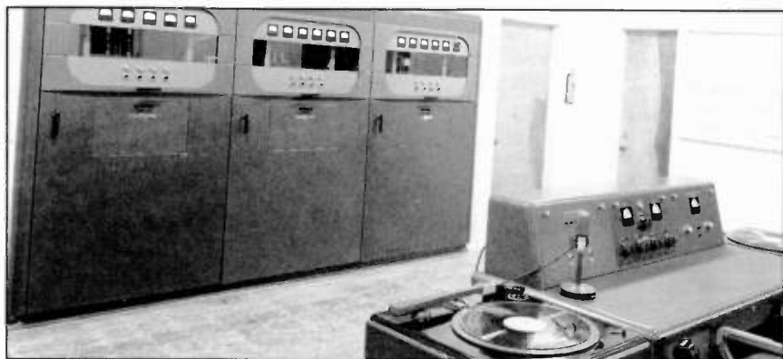
Collins 10 kilowatt FM broadcast transmitter and disc jockey console, typical of equipment installed at KCRG-KCRK in Cedar Rapids and many other radio stations after World War II.
