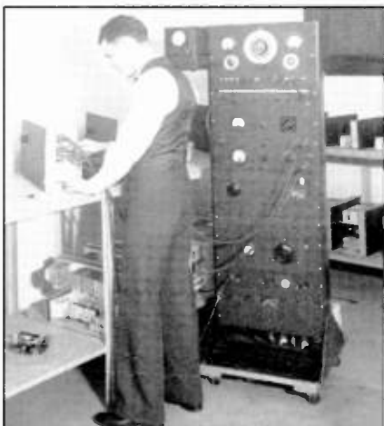
W.F. (Bill) Stewart testing amplifiers, part of the Collins line of commercial broadcasting products of the 1930s. Stewart joined the company in 1935.
