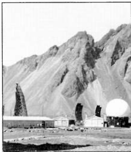
A DEW Line installation, with radar dome and Collins-built billboard type troposcatter antennas.
