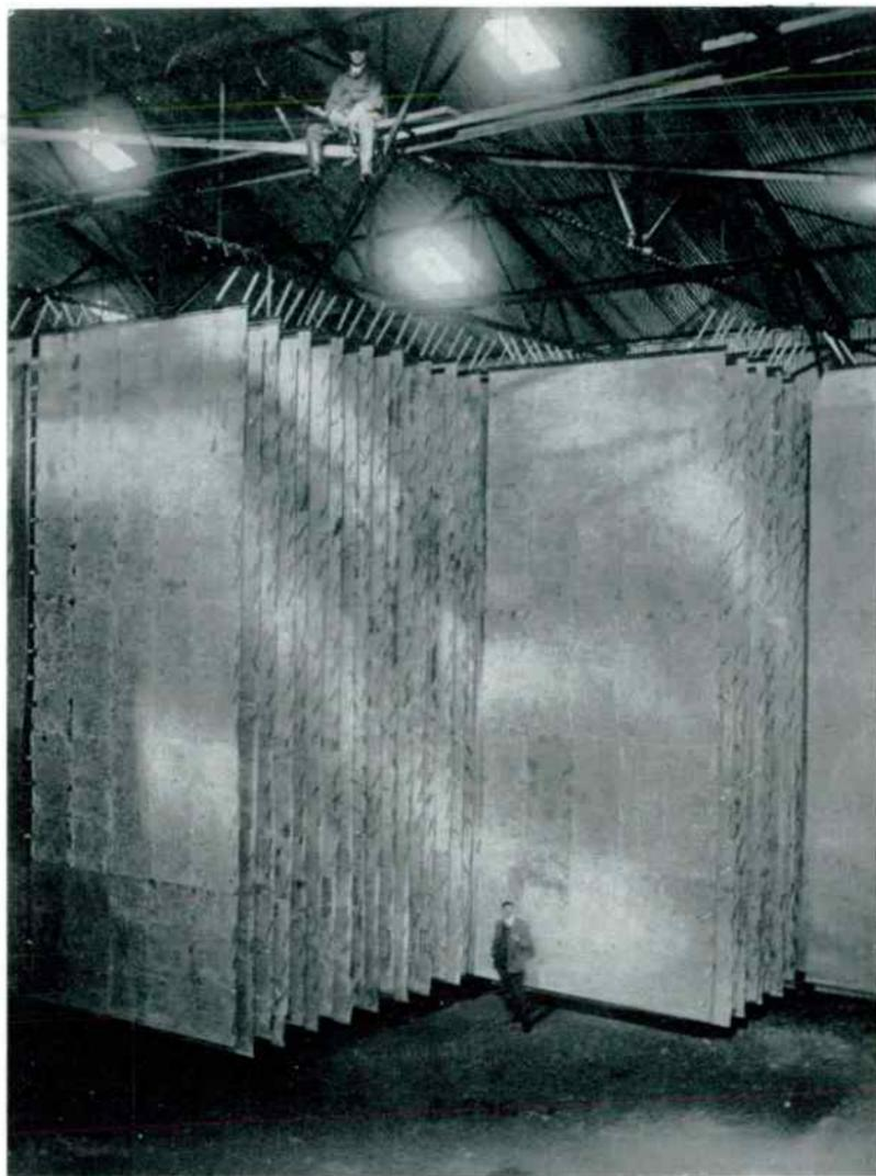
15 *The main capacitor at the Clifden station under construction, about 1906. The generous air space between the galvanized steel sheets ensured reliable operation at about 80,000 volts, but 1,800 sheets were needed to attain the required capacitance of 1.16 microfarads*
