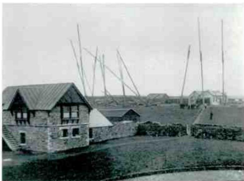
to copy; though each mast was stayed against radial movement, its only tangential constraint came from horizontal wires tying it to its neighbours. Vyvyan's objection was over-ruled, and no heed was taken of his subsequent warning, in August, that the aerial he had built at Cape Cod was dangerously distorted by no more than a stiff breeze.
