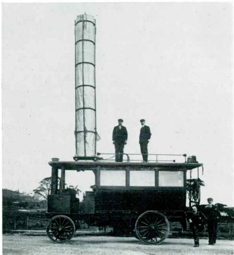
6 An experimental mobile station, 1901 ; the aerial was hinged back to lie horizontally when the vehicle was on the move. Marconi and Professor Fleming can be seen at the rear of the vehicle
