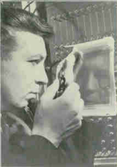
An RCA computer scientist inspects an experimental memory device which can store a quarter-million bits of information when immersed in liquid helium.
