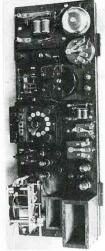
Fig 45. Lodge electrolytic detector (1910); Lodge-Muirhead experimental equipment.
