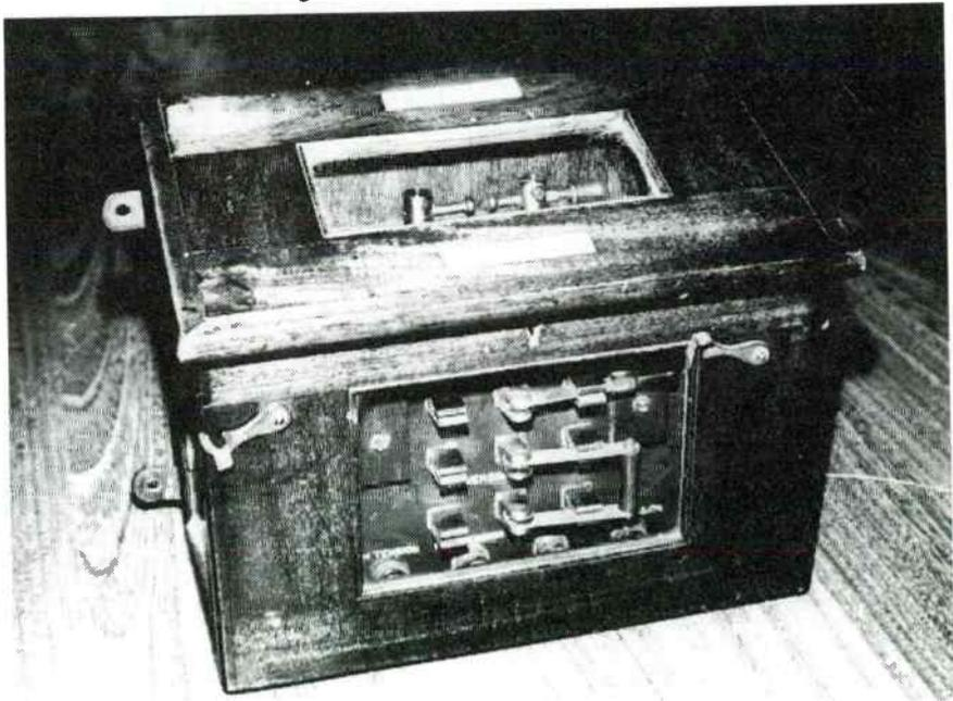
Fig 47. The Lodge igniter for motor cars.
