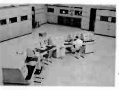
A view of TWR's transmitter master control at Monte Carlo. Located here are two 100,000-watt shortwave transmitters leased from Radio Monte Carlo. TWR transmits on medium wave during prime evening hours and on long wave to France in the early morning.
