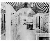
FEBC overseas transmitters located at Bocaue, Philippines. Equipment includes six 50,000-watt transmitters, one 10,000-watt transmitter and one 100,000-watt transmitter.
