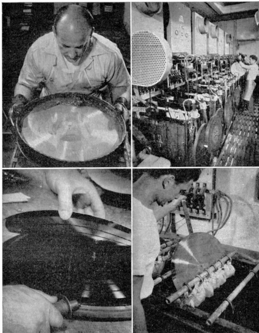
FIG. 21. Making a transcription. This picture series was taken in Recorders Labs, Limited, a Hollywood transcription processing company which makes pressings for leading transcription companies. Upper left , silver is deposited on the original instantaneous transcription. Upper right , copper-plating the original transcription. Lower left , separating the original transcription from the metal master. Lower right , electroplating the metal master with nickel. ( Recorders Labs, Limited. )
