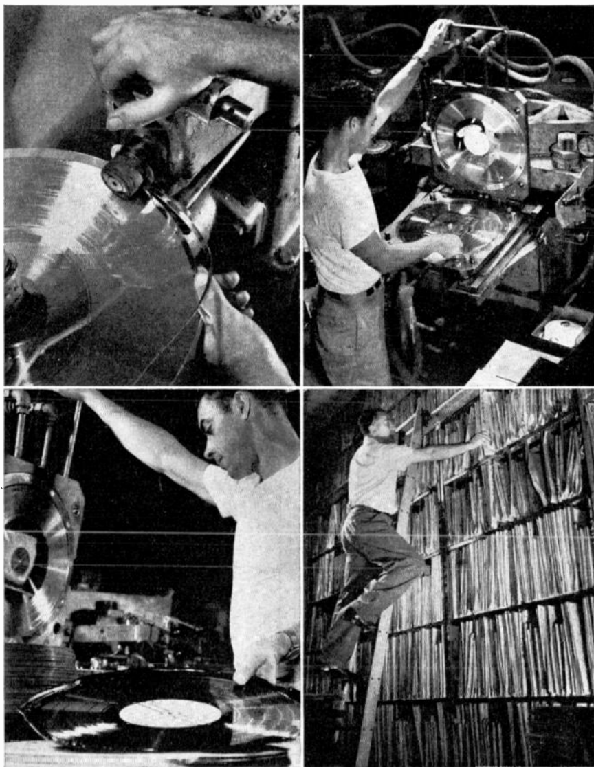
FIG. 23. Making a transcription. Upper left , shearing the stamper to size. Upper right , placing a vinylite "biscuit" in the stamper. Lower left , taking an untrimmed transcription (pressing) off the press. Lower right , filing the metal master, the metal mother, and the stamper plate. ( Recorders Labs, Limited. )
