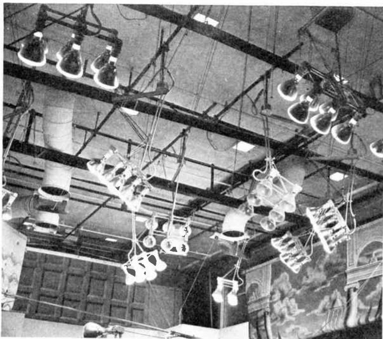
FIG. 16.—Lighting units are mounted on a grid attached to the ceiling. Each unit may be rotated and tilted at any angle by remote control.
