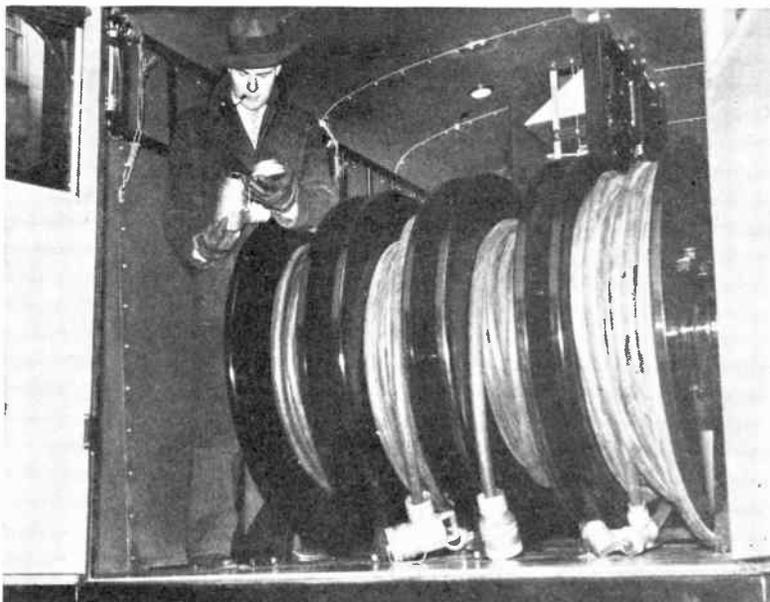
FIG. 47.—Reels of cable in the rear of the transmitting truck.
