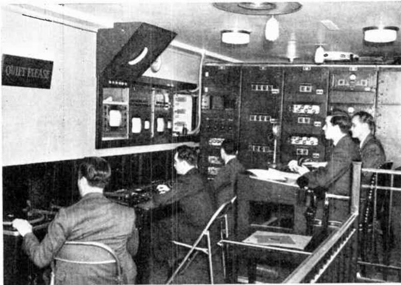
FIG. 18.—The master control room overlooking the live-talent studio. The three men in the front row, from back to fore, are; the video engineer, the sound engineer, and an engineer handling music and sound-effects turntables. Behind these three are the technical director in the back and the program producer in the fore.
