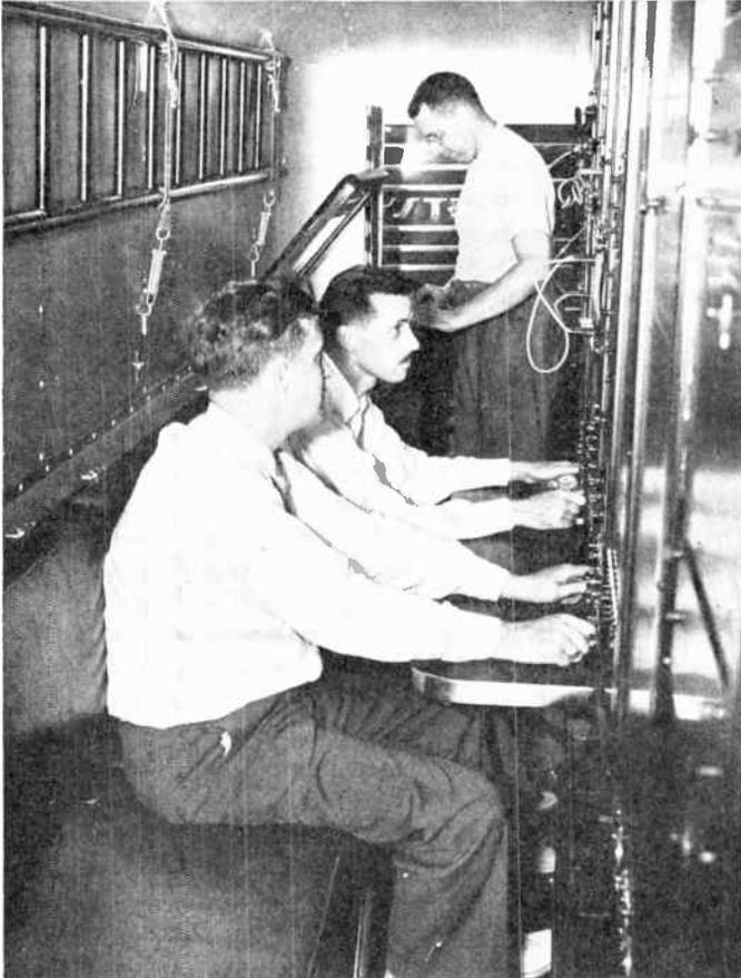
FIG. 50.—Another view of the control position, showing the audio and video engineers at work. In the rear, an engineer is monitoring the picture on a home-type receiver.
